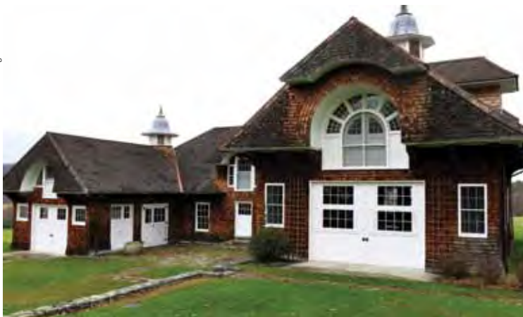
Located in a converted horse stable, the print studio is housed in the left wing, while the painting studio is on the right in the former carriage barn
